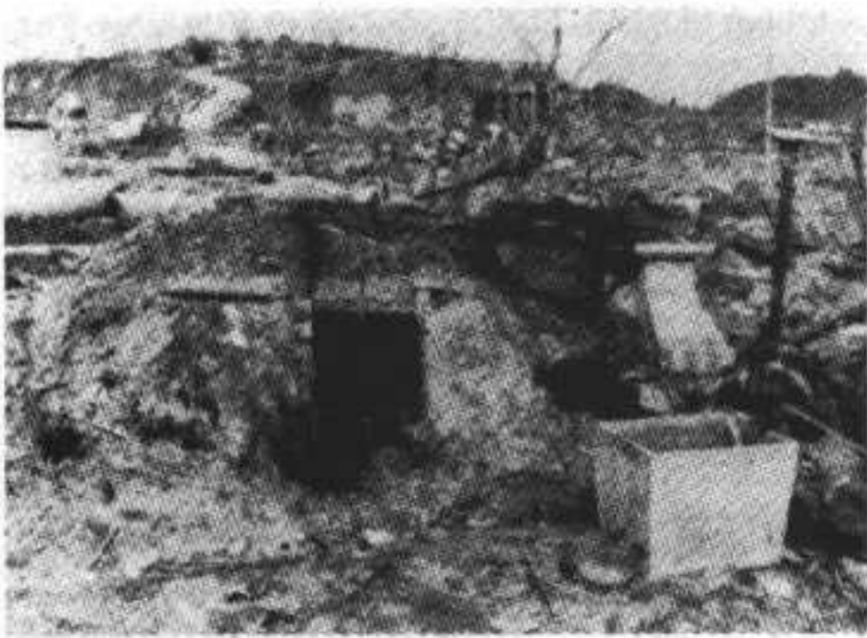
Fig. 1.5. Undamaged earth-covered family shelter in Nagasaki.
