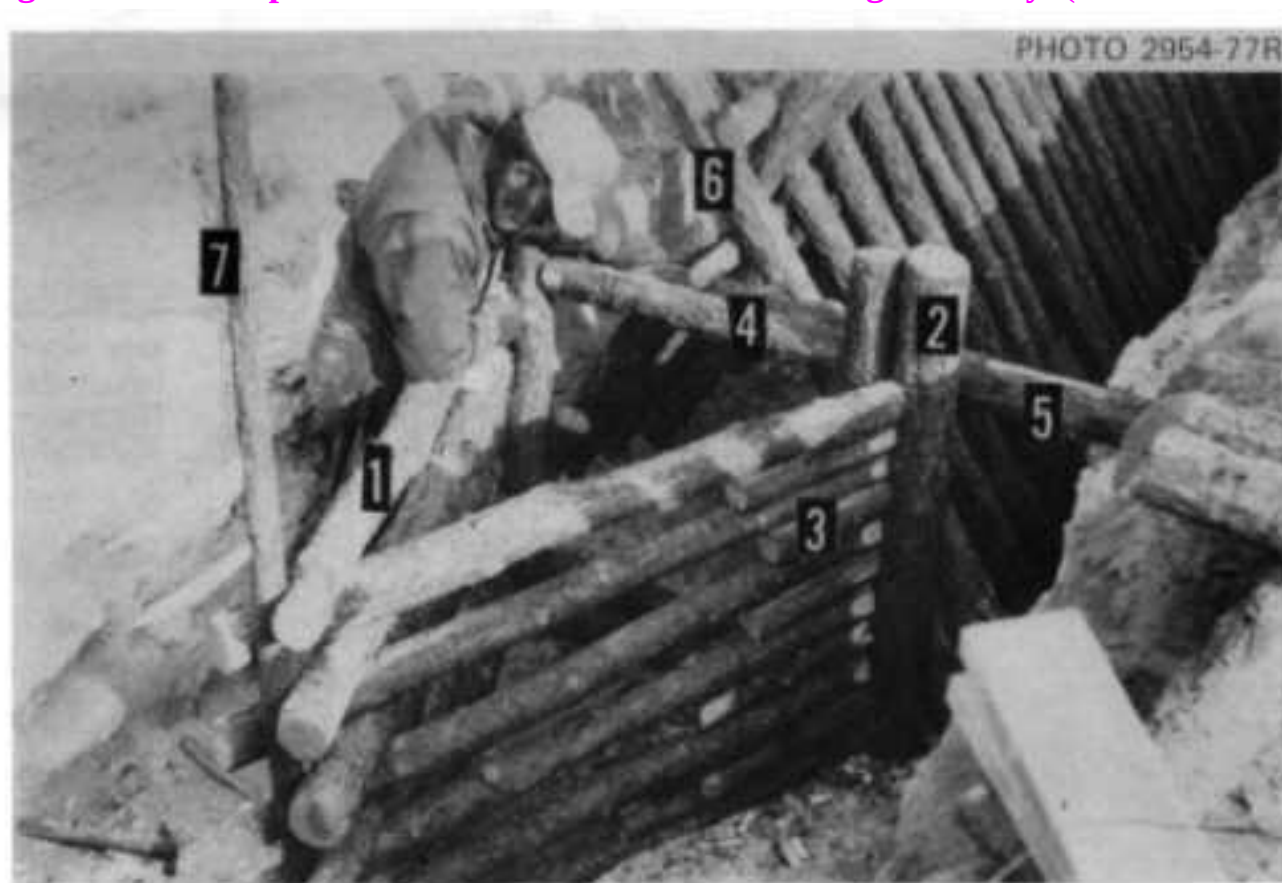
Fig. D. 10. Uncompleted lower section of a vertical triangular entry. (Photo 2954-77R)
